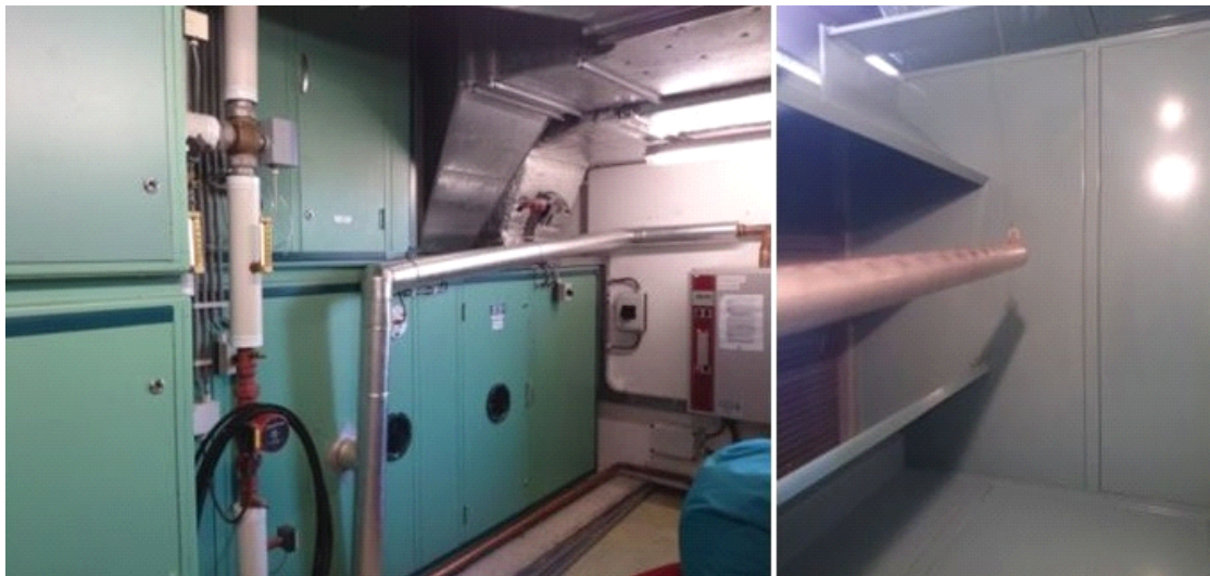
Figure 13 Air Handling Unit and steam pipe
