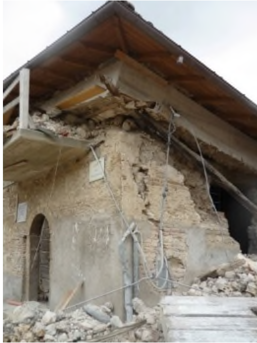
Figure 4 In L'Aquila, the heavy substituted roof caused the crumbling of the walls of the level beneath it [10]
