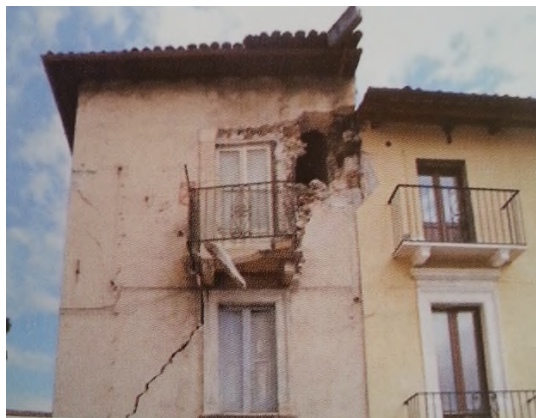
Figure 5 damage caused by the adjacent building [20]
