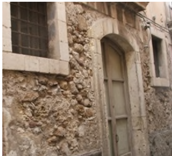
Figure 3 poor quality masonry in Ortigia
